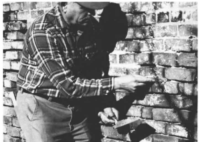
The author repoints a brick wall.
