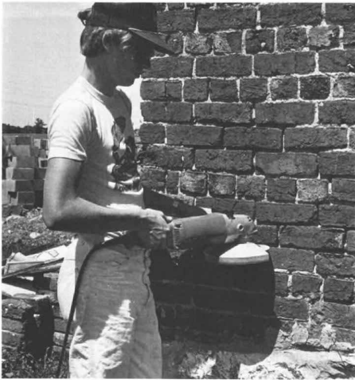
Removing mortar joints —Mortar joints can be removed using a power grinder (A), but it takes a skilled operator to avoid damaging the brick. To remove the joints by hand, use a plugging chisel (B, top) specially shaped for the job. The mason's all-purpose chisel (B, bottom) has other uses. Cut the joint out squarely (C). Brush out mortar particles with a soft-bristled brush (D). Use the same brush to dampen the joint before repointing.
